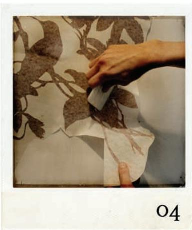
*04 . Using the scraper, firmly press the sticker to the wall. Start at the centre and smooth towards the edges to drive away air bubbles.*
